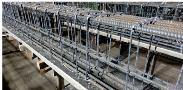
Figure 2. Reinforcement binding.
