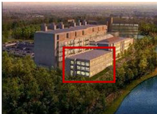
Figure 5. Overview of Target Building A.
