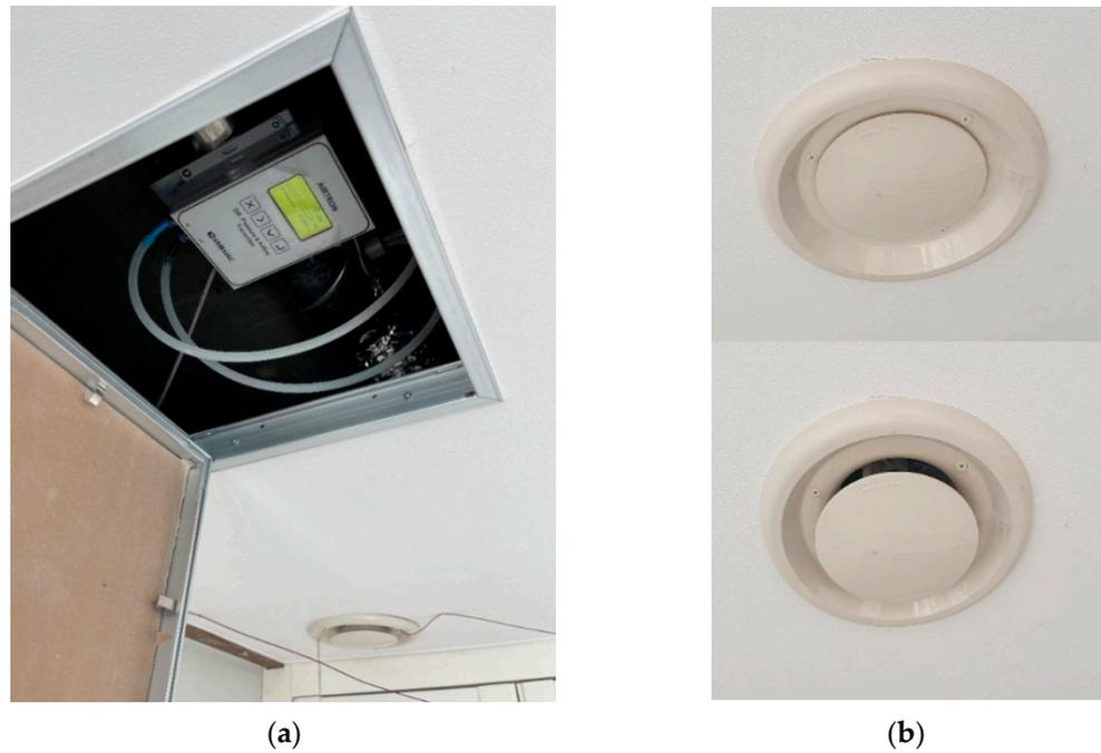
**Figure 2.** The variable air volume controlling system: (a) flow metering system (FMS); (b) motor diffuser closed (upper) and opened (lower).
