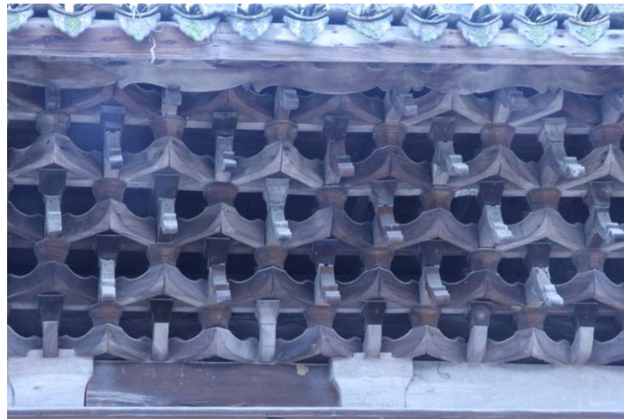
Figure 10. The door covers of a traditional building in central Jiangxi.
