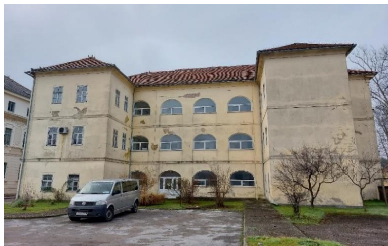
Figure 3. North-east facade of case study building.
