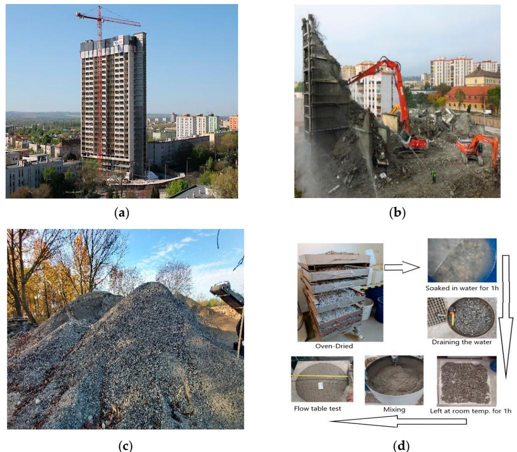
**Figure 2.** (a) High rise building that was the source of recycled aggregate ; (b) Demolition technique; (c) Stored debris ; (d) Steps for partially saturating the recycled aggregates.
