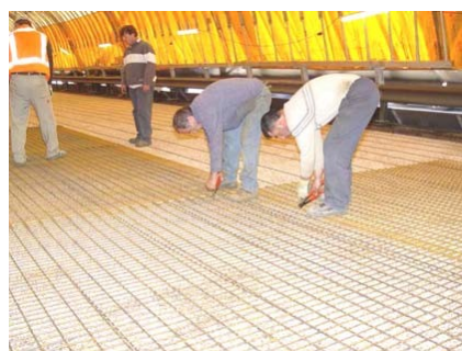
Figure 7. Deck replacement of Galand Bridge using glued UHPC layer.
