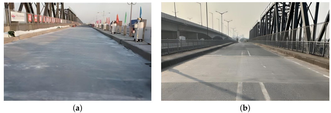
Figure 8. Mafang Bridge using steel–UHPC composite deck: (a) Under construction; (b) After 12 years in service.
