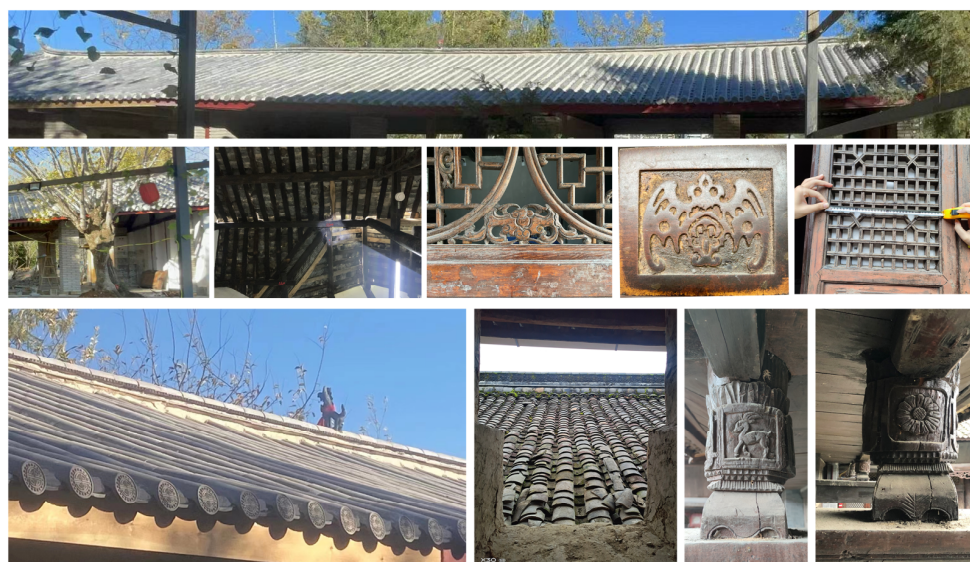
Figure 4. Site status (tiles, wadang (eaves tile), grid, auspicious animal, wood carvings, etc.).
