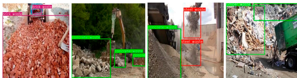
Figure 9. Examples of true positive prediction brick, concrete, steel, and timber wastes.
