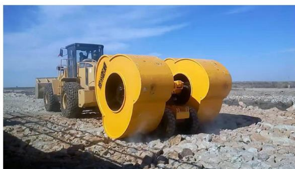
(c) Use of manufactured aggregate for dam construction
