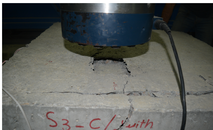
Figure 6. Crushing in the concrete of specimen S3-C.
