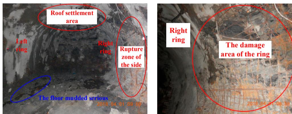
**Figure 4.** Deformation of 2-2 medium-coal roadway.
