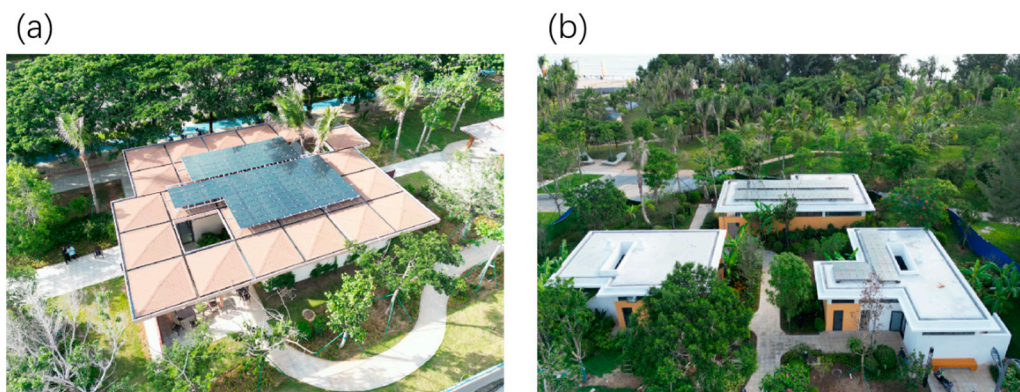
Figure 5. Top view of zero carbon building project. (a) City block post station. (b) Coastal city post station.
