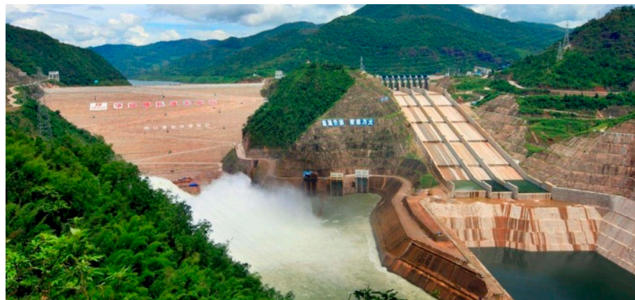
Figure 7. Scene of Nuozhadu Dam.
