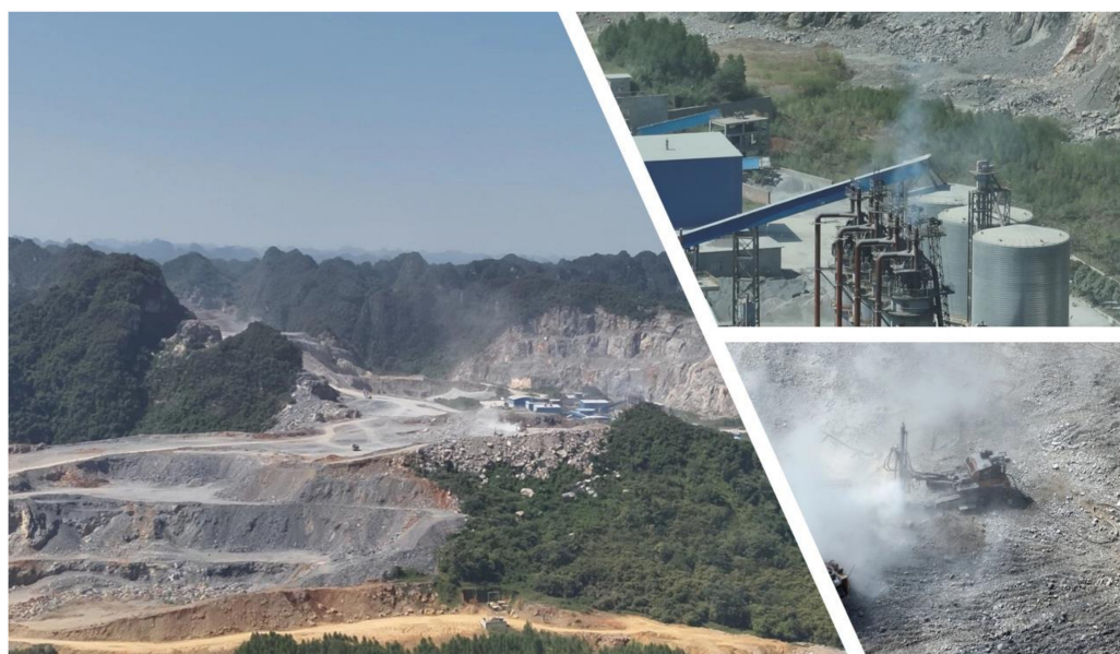
Figure 1. Mining and production sites of cement factory in Guangxi province, China.
