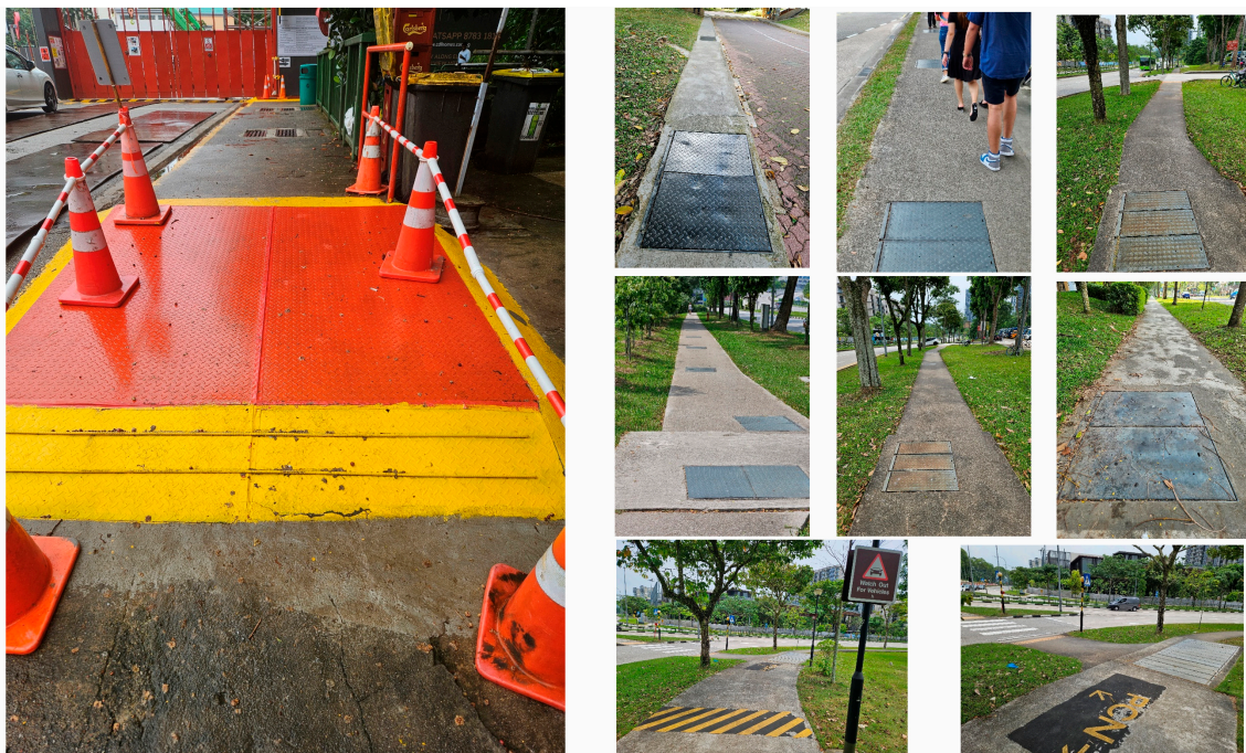
Figure A2. Metal coverings on ramps and manholes.
