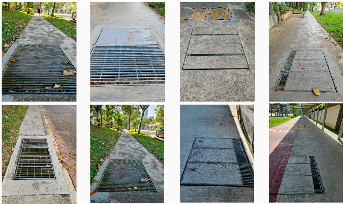
Figure A3. Drainage metal grills.
