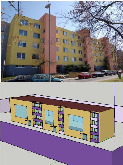
Residence Building RB1—1976
