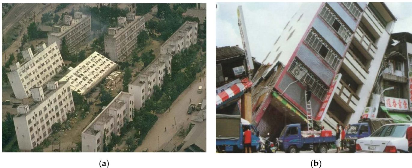
Figure 1. Building collapses due to earthquake liquefaction. (a) Niigata earthquake in Japan in 1964, (b) Taiwan earthquake in 1999.
