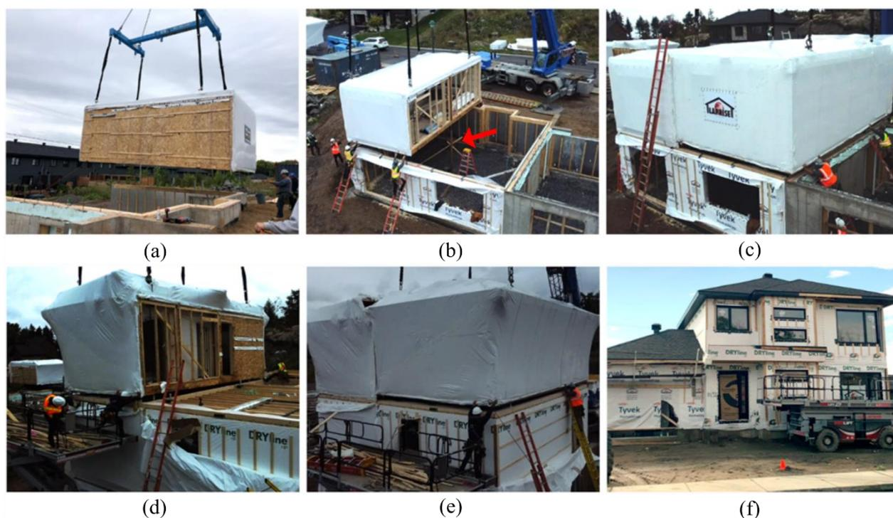
**Figure 7.** Overview of the on-site assembly process of the full-scale experimental project: (a) testing of the lifting equipment; (b) rear view of module 1 installation; (c) rear view of module 2 installation; (d) rear view of module 3 installation; (e) rear view of module 4; and (f) façade of completed assembly.
