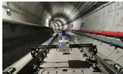
Figure 3. Tunnel inspection vehicle site survey map.
