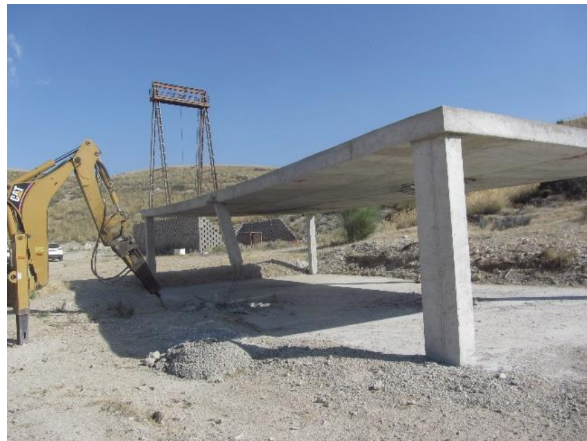
Figure 3. Two-span structure: demolition of central column using a pneumatic hammer.
