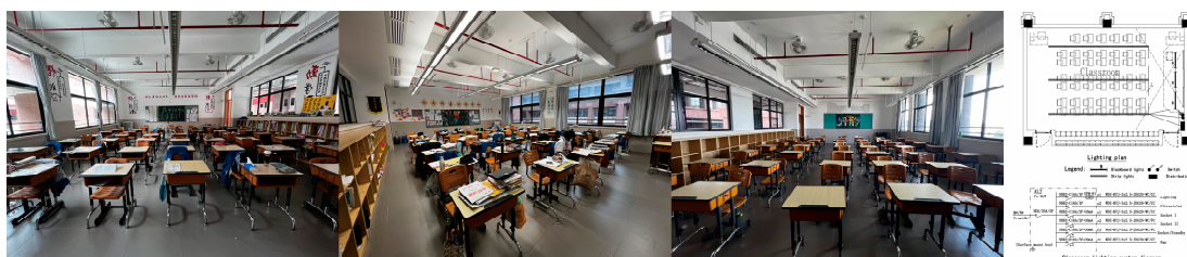
Figure 7. Classroom lighting arrangement. The three classroom lighting systems are all arranged in the same manner, with three strip lights evenly spaced in the classroom and blackboard lights in parallel at the front.
