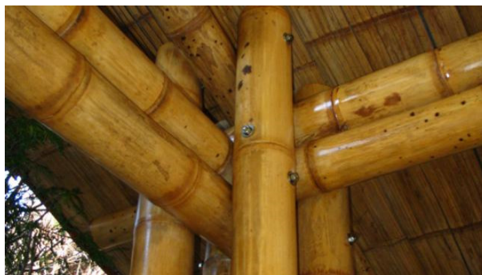
Figure 13. Bolted connections [78].
