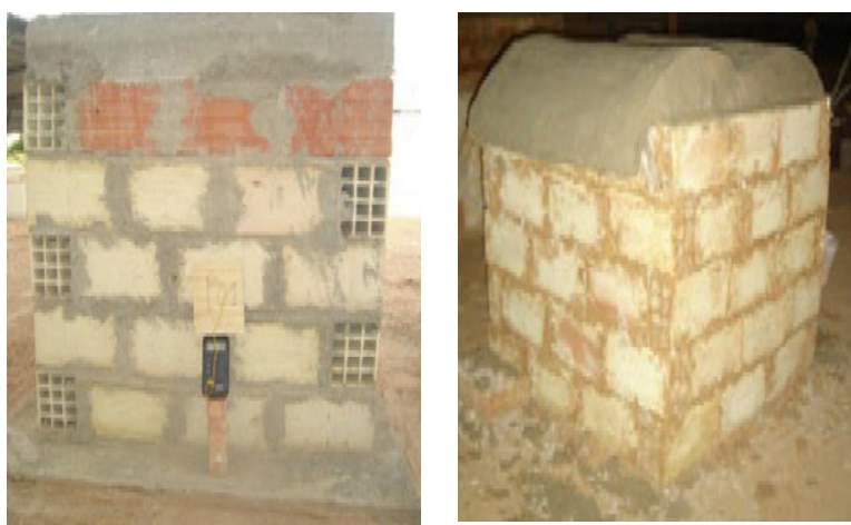
Figure 13. Wall construction and testing with varieties of block materials [76].
