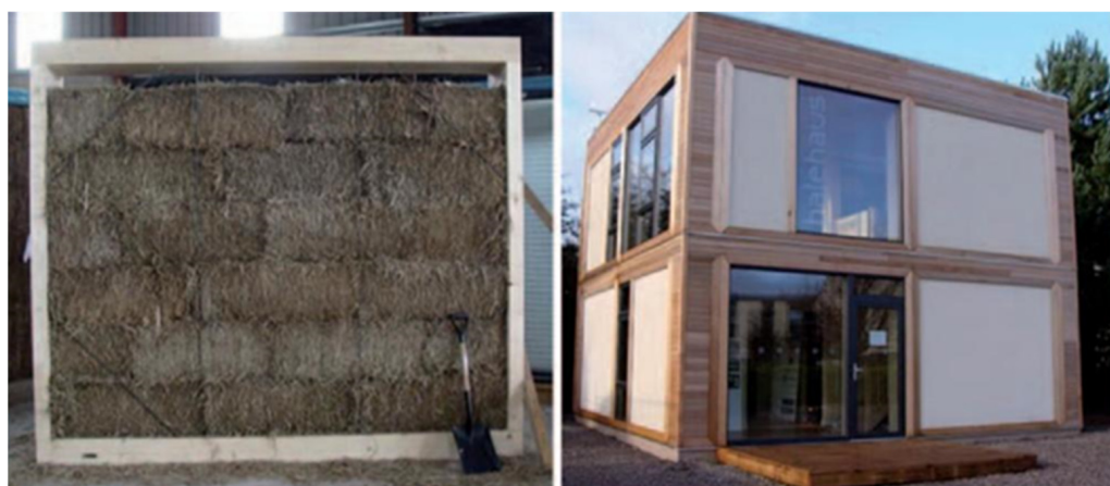
Figure 8. ModCell panel (left) and the complete prototype house at the University of Bath campus (right).
