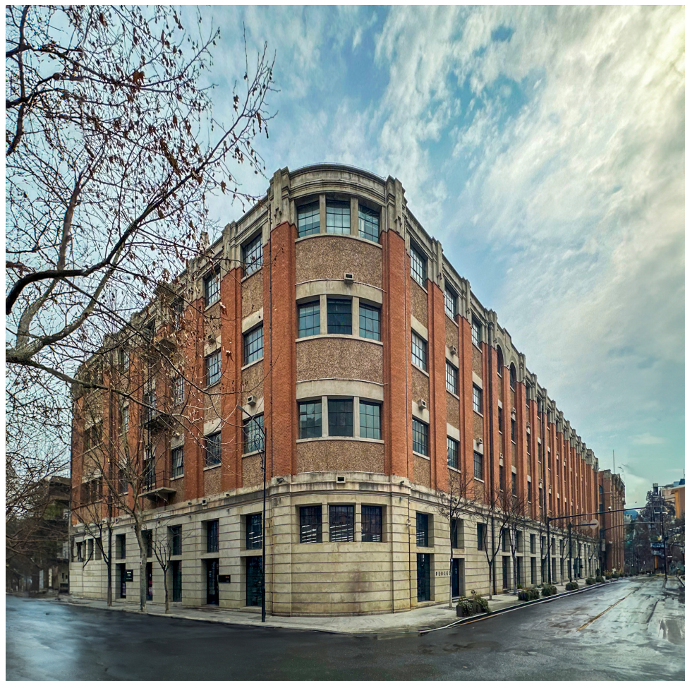
Figure 8. Photos of the site after rehabilitation of the Pinghe Packing Factory.
