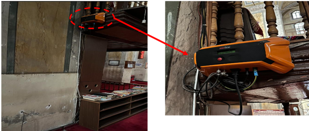
Figure 9. Installation of the capillary rising damp treatment device.
