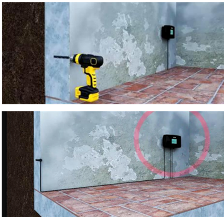
Figure 3. First stage of installation of the capillary moisture treatment device [41].
