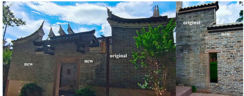
Figure 5. Picture of the restored ancient building wall in Qi Li Ancient Town.
