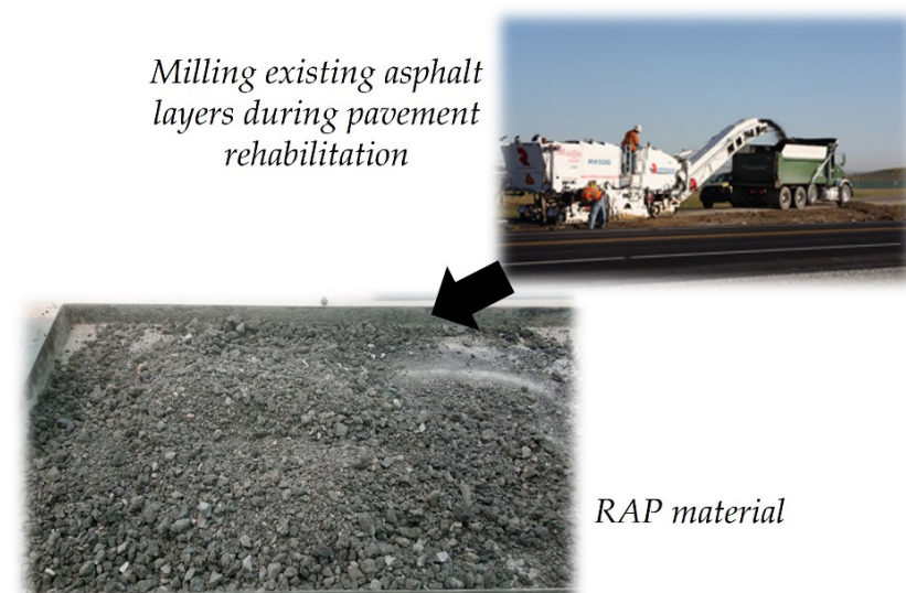
Figure 6. Process to retrieve RAP.
