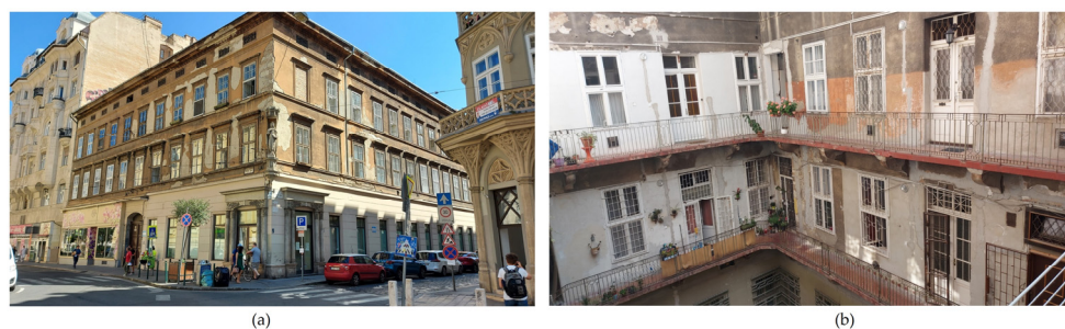
Figure 2. Street façade (a) and courtyard façade (b) of a typical old residential building in Budapest.
