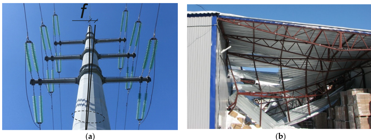
Figure 13. Cases of load identification by displacements: power line supports (a); roof trusses after an accident (b), f is the deviation of displacements caused by the uncertain load; f - upper point deflection.
