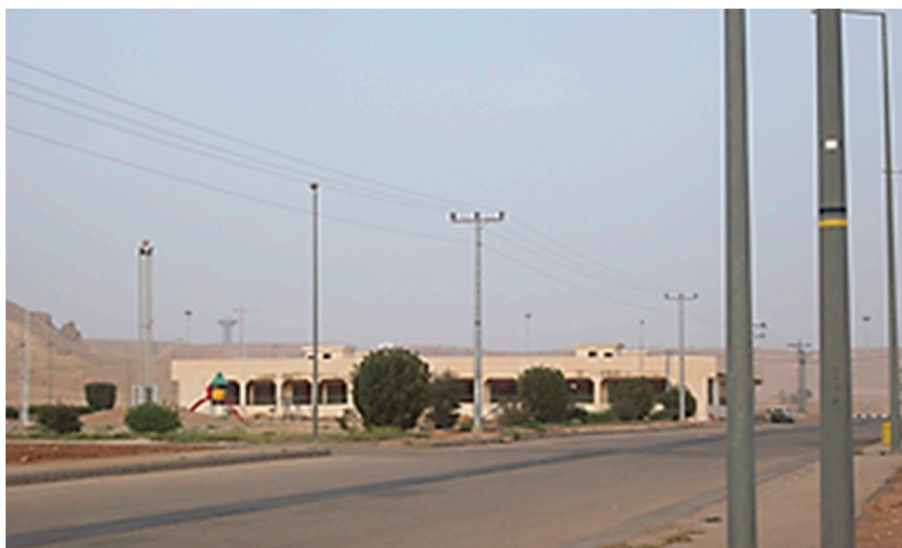
Figure 1. A market building affected by expansive soil in Al-Ghatt town.
