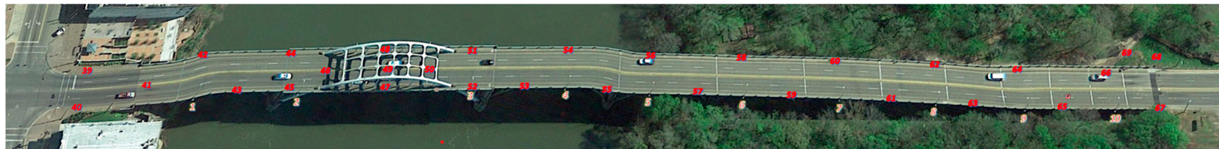
Figure 10. Planned scanner locations on the bridge's deck.
