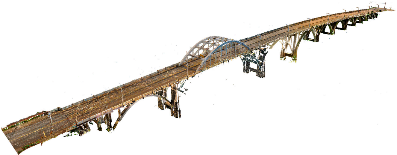
Figure 11. Registered point cloud of the whole bridge.
