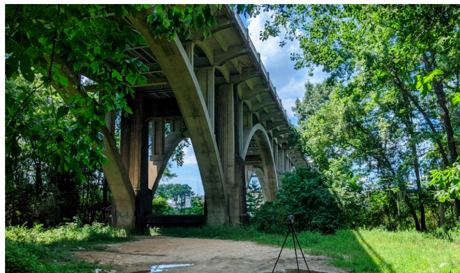
Figure 7. Dense vegetation around the bridge.
