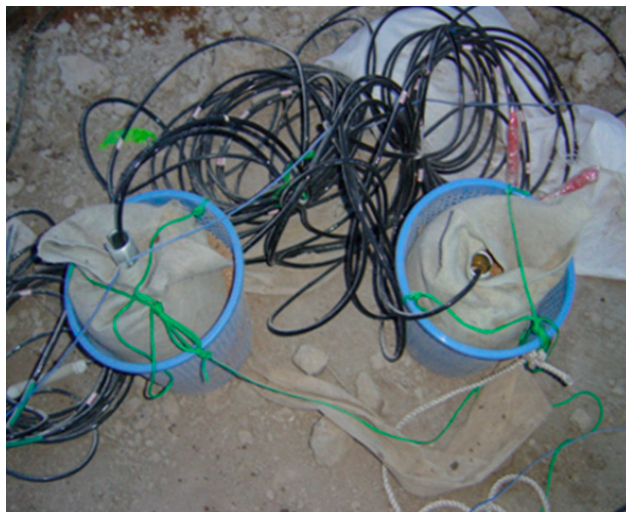
Figure 12. Installation of pore water pressure gauge.
