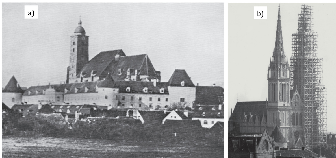
Figure 1. Zagreb Cathedral: (a) before the earthquake of 1880 [1], (b) restoration of the southern bell tower, 1938–1940 [2].
