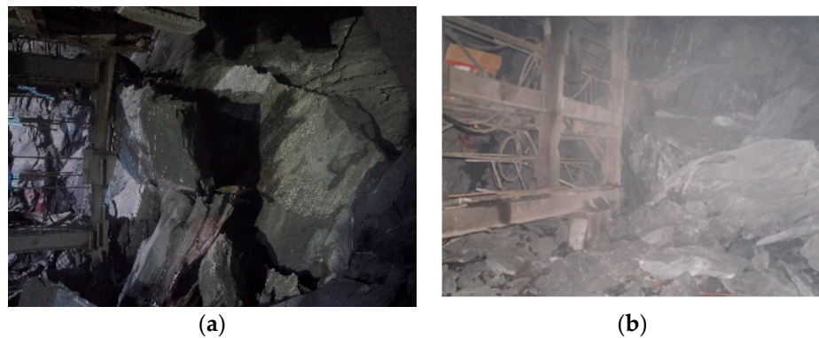
Figure 4. Right line of Ping'an Tunnel strong rockburst outbreak site: (a) Strong rockburst (YD8K171+805). (b) Strong rockburst (YD8K171+946).
