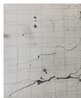
The lower right part of the wall
