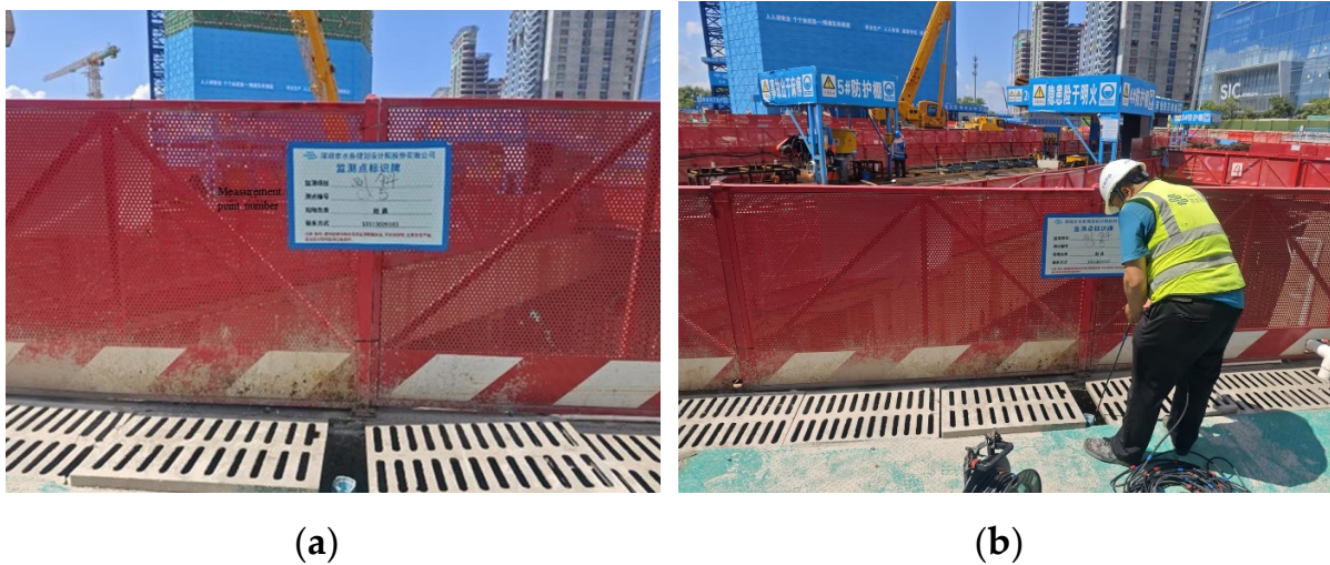
Figure 13. (a) Pictures of CX-5 monitoring point. (b) Monitoring personnel on site.
