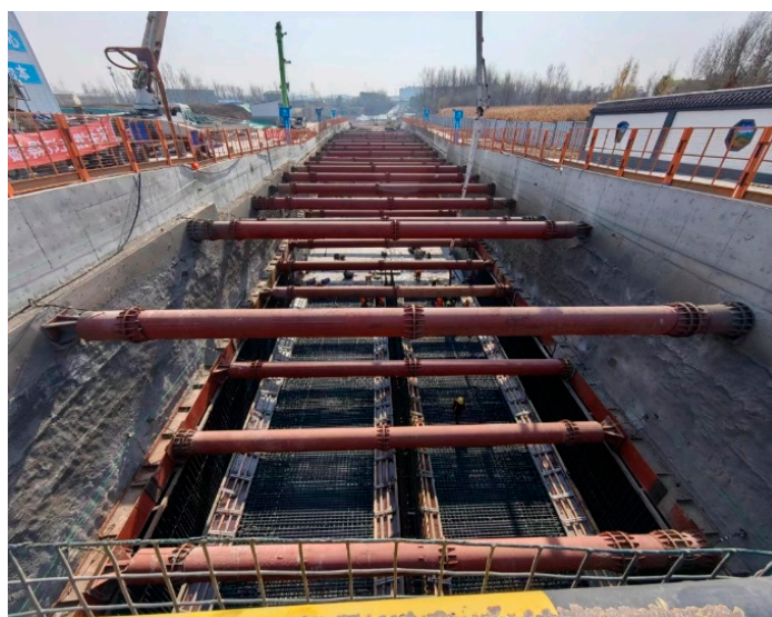
Figure 3. Arrangement of steel supports.
