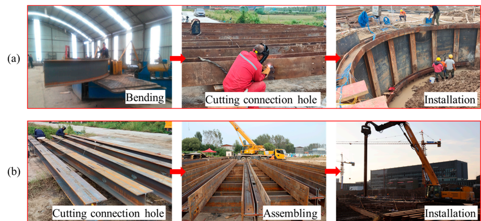
Figure 3. Prefabrication on the PRSS: (a) waling; (b) supporting piles.
