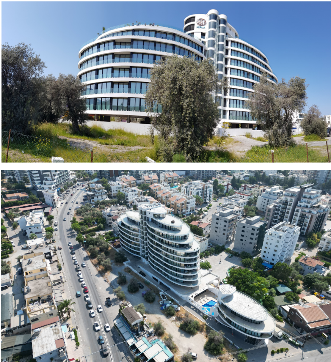
Figure 6. Perla Building (Source: Author).
