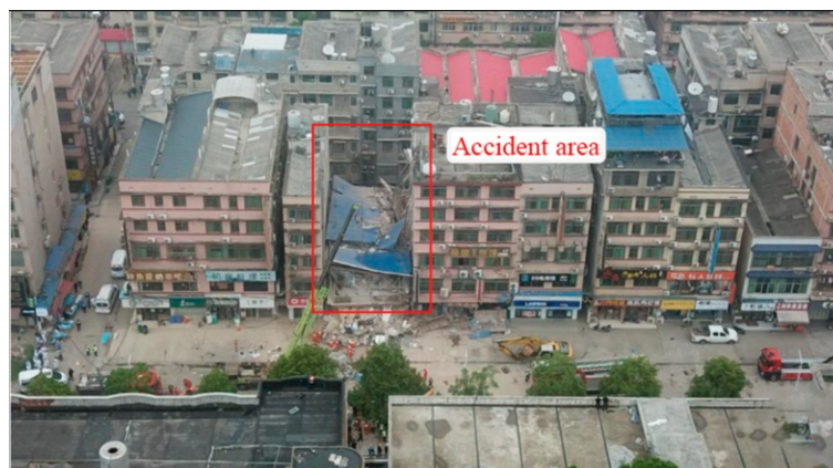
Figure 1. Photo of the collapsed building, Changsha, China (Reprinted/adapted with permission from Ref. [7]. Wang et al., Int. J. Environ. Res. Public Health , published by MDPI, 2023).
