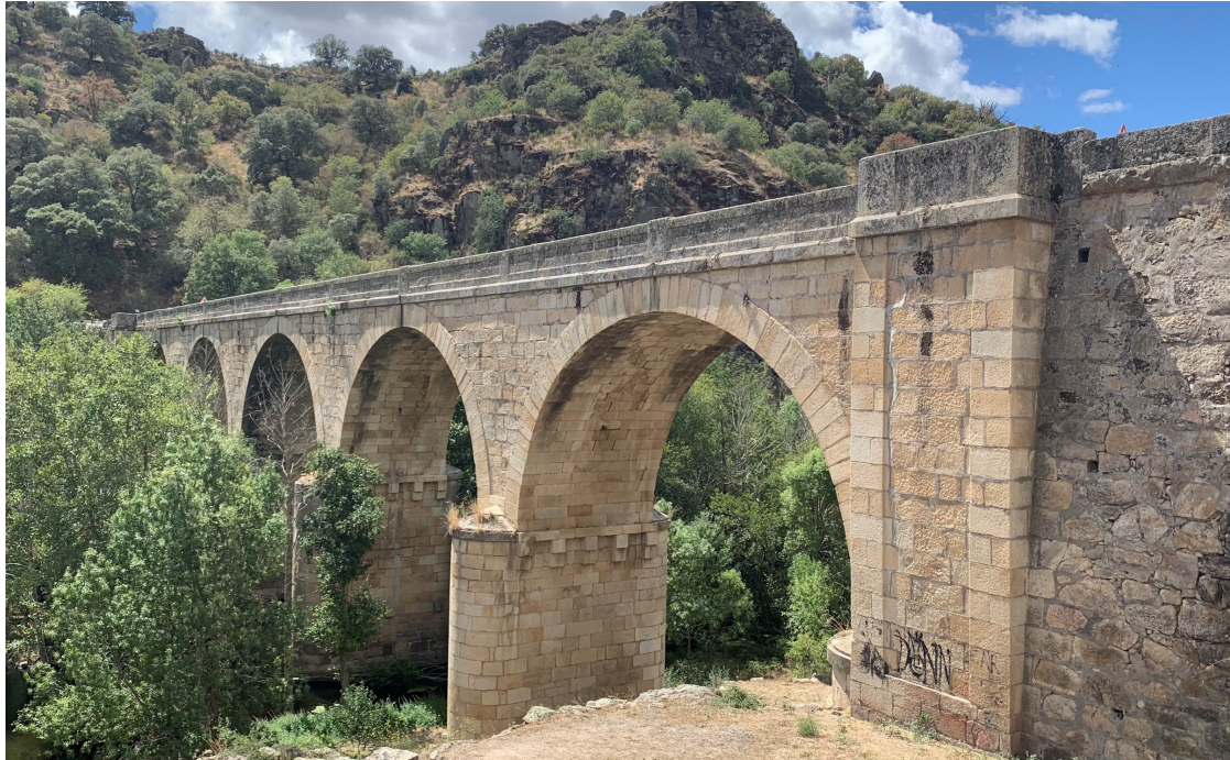
Figure 10. Image taken from the northern abutment, on the Zamora side, of the San Lorenzo Bridge (photo by the author).
