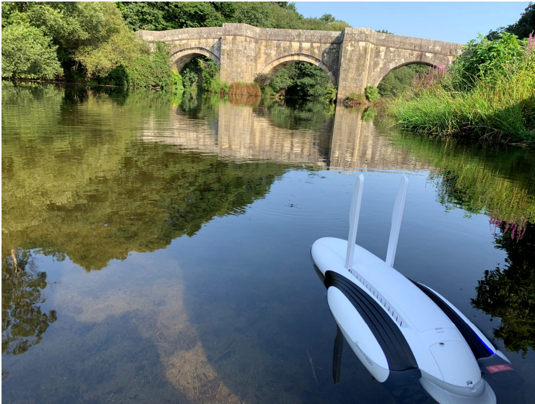
Figure 17. Underwater drone moving along the Xallas River, approaching the downstream side of the Brandomil Bridge (photo by the author).
