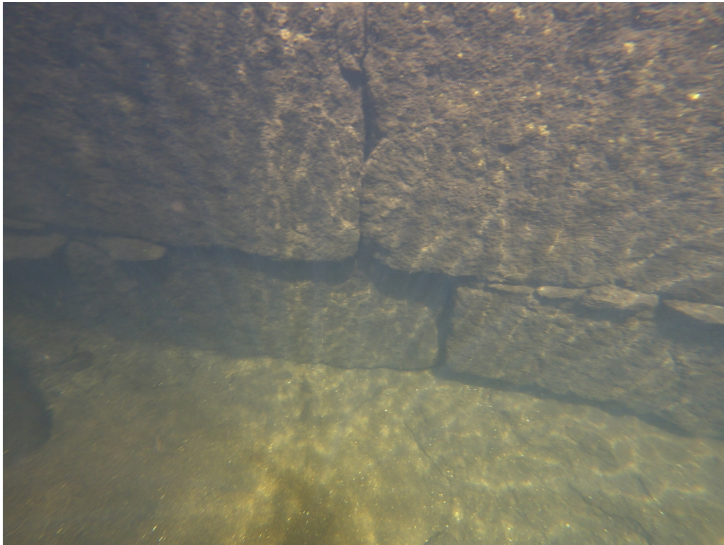
Figure 14. Underwater drone image showing the status of a fragment of the lower part of the pile inspected in the position of Figure 11 (photo by the author). The granite ashlars and the fixing slabs can be seen in the image.
