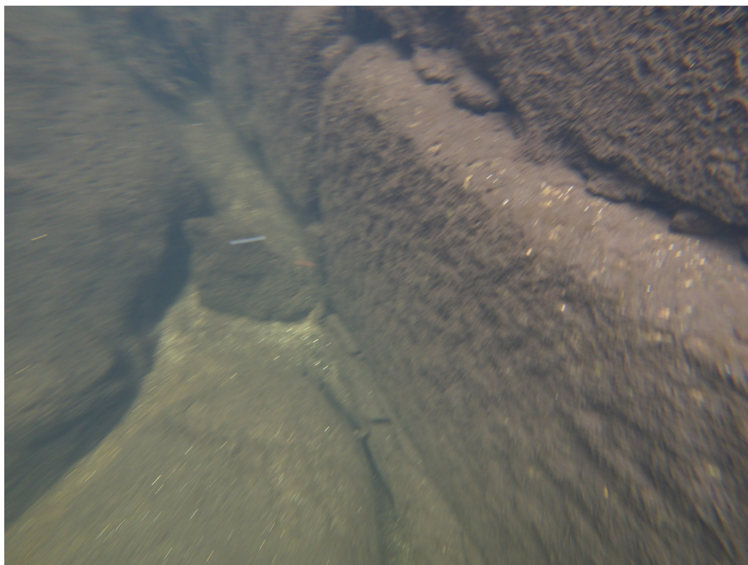
Figure 15. Condition of another fragment of the lower part of one of the inspected piles, in an image captured by the underwater drone (photo by the author). The stone elements on the river bottom, around the base of the piles, can be seen in this photograph.
