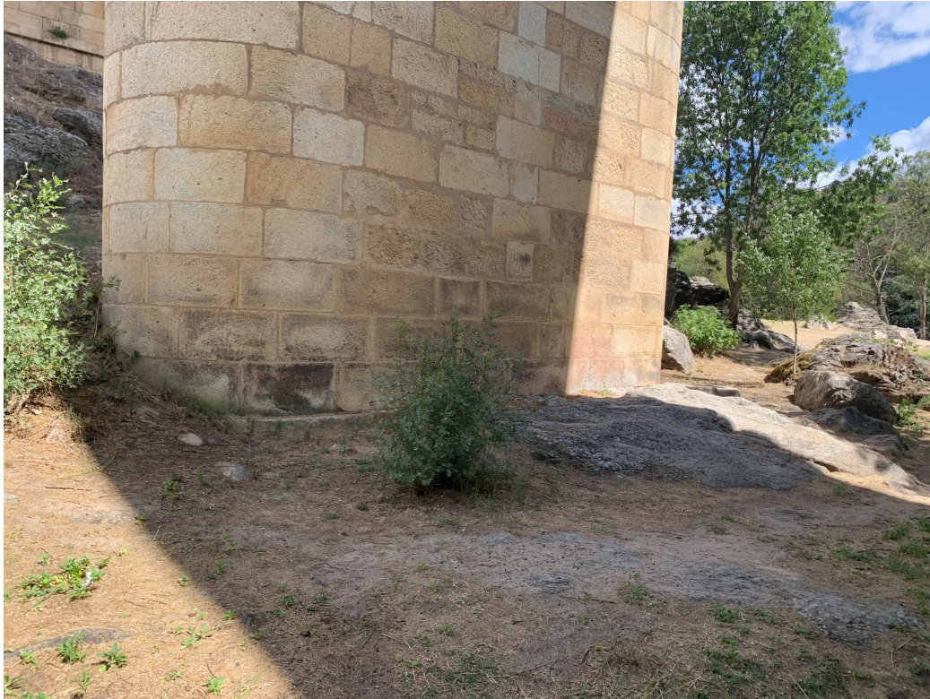
Figure 13. Another view of the pile shown in Figure 12, with the northern abutment in the background (photo by the author). This photo also served to give an idea of the foundation of the bridge elements, as not all of them were visible.
