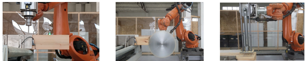
Figure 1. The proposed robotic timber construction process.
