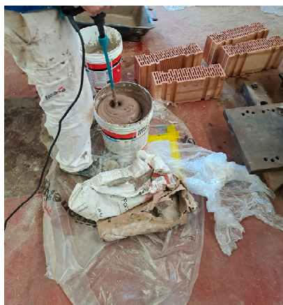
Figure 2. Preparation of Porotherm special mortar.
