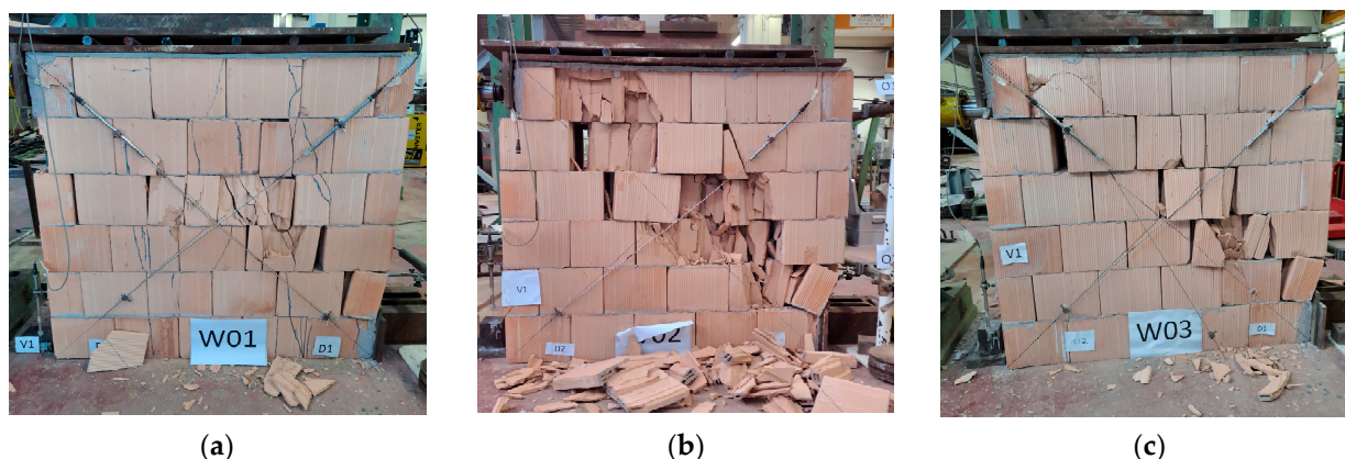
Figure 13. Collapsed state of W01 (a), W02 (b) and W03 (c).
