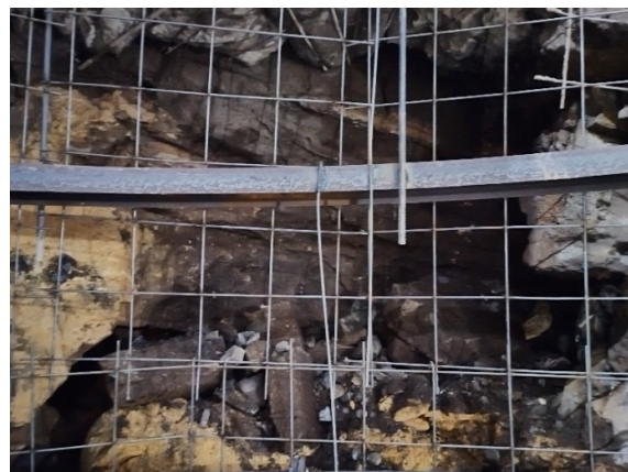
Figure 3. Karst development pattern in the vertical shaft.
