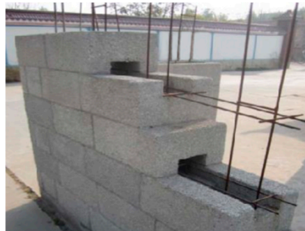
Figure 1. Grid shear wall with insulated masonry.
