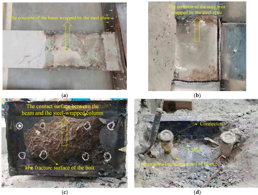
Figure 15. Failure phenomenon of the core area: (a) concrete of the beam near the core area; (b) concrete in the core area; (c) cross-section of bolts after the test; (d) experimental phenomenon of the connector.
