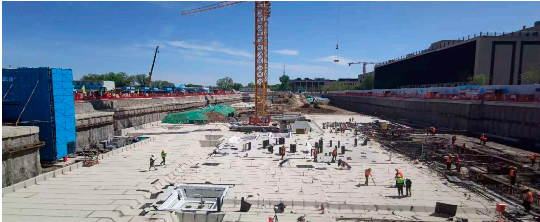
Figure 11. The excavation construction site of the project.
