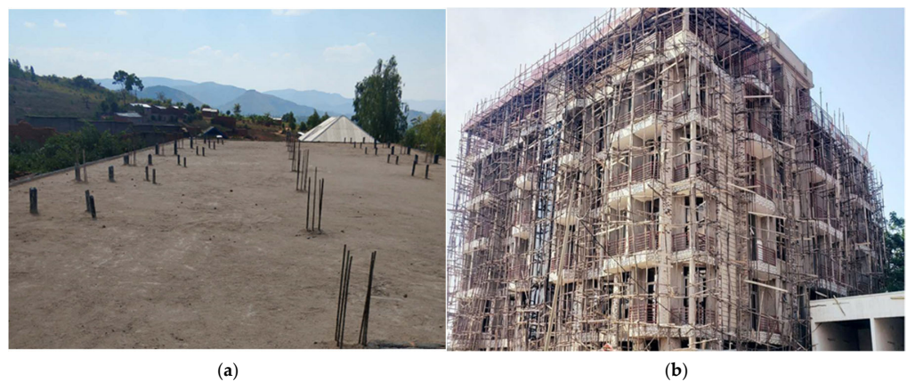
Figure 8. Typical example of a delayed project due to delayed material delivery caused by weather conditions (a) and abandoned project due to late delivery of materials caused by weather, low bid price of a contractor, and ineffective road infrastructure (b).
